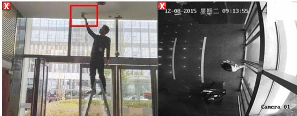
Passenger flow in horizontal direction (wrong)
