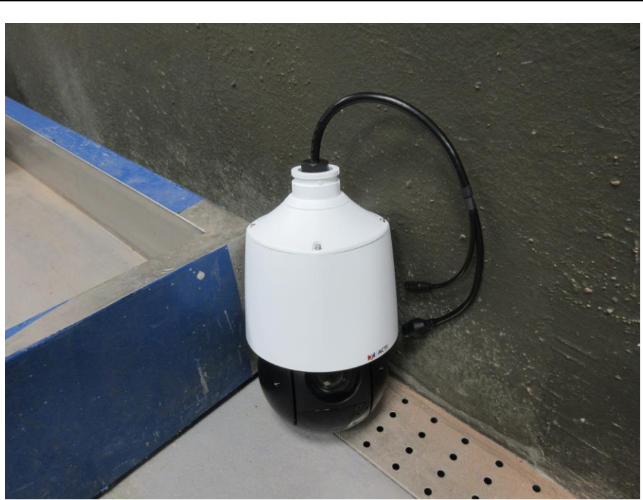
Photo of EUT before water test
